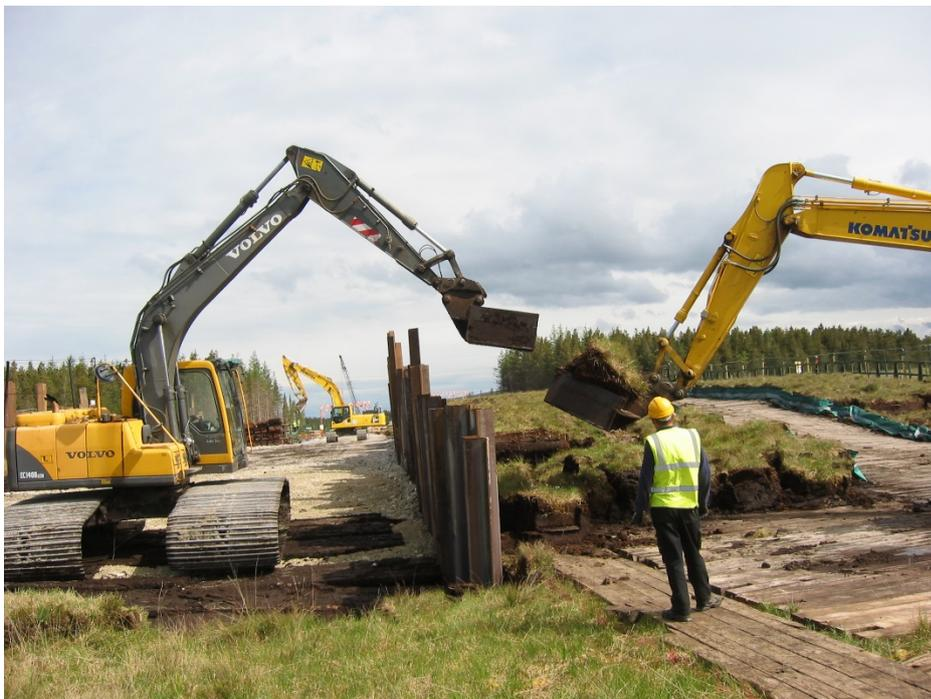
iii. Turve storage on bogmats (on RHS of sheet piled haul road and trench section on left)
