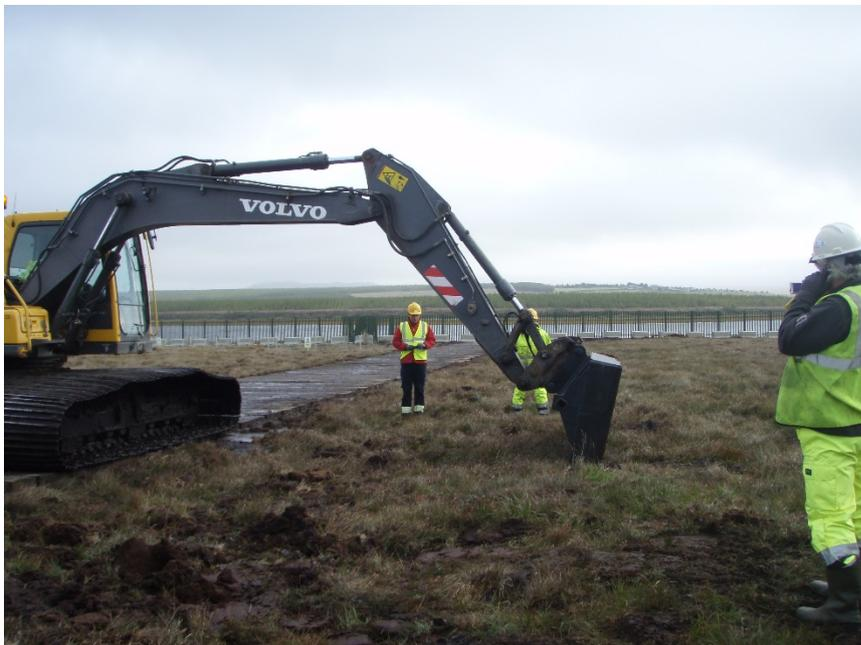
**2b. Transfer bucket + turve to back of low impact truck**
