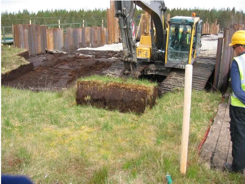
**ii. Then transferred from the 'lifting' machine's bucket to the machine placing turves on bogmats in the adjacent storage area – required excellent driver coordination and care.**
